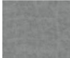
Broken Concrete | Grey
